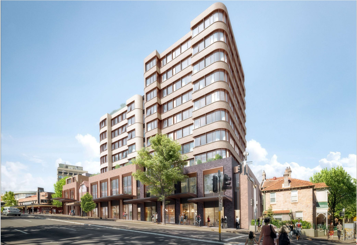
The 3D model illustrates how the stepped streetwall height enhances the slender, vertical tower proportions (PTW December 2021).
